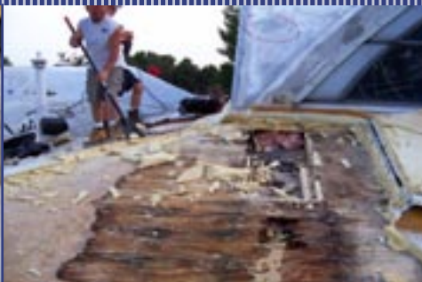
Tear off of deteriorated roofing material.
