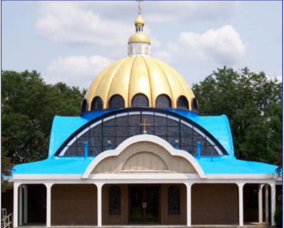
This roof received a 10 year renewable manufacturers warranty.
