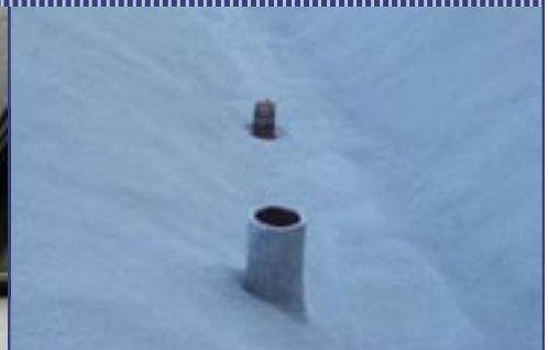
"After" picture of drain and vent stack in valley.
