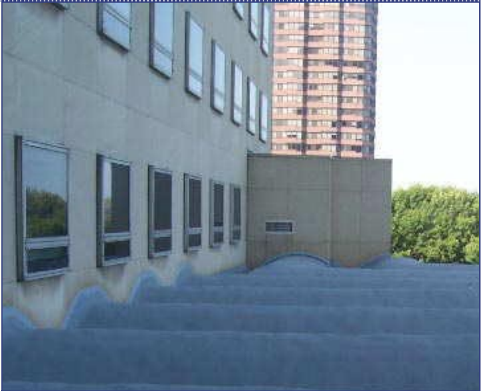
This scalloped hospital roof received a 10 year manufacturers warranty.
