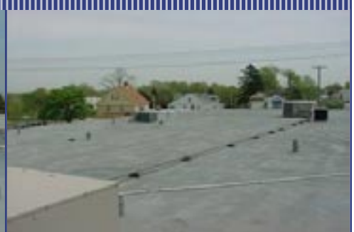
Ceramic granules are embedded into the final silicone top coat for added protection.
