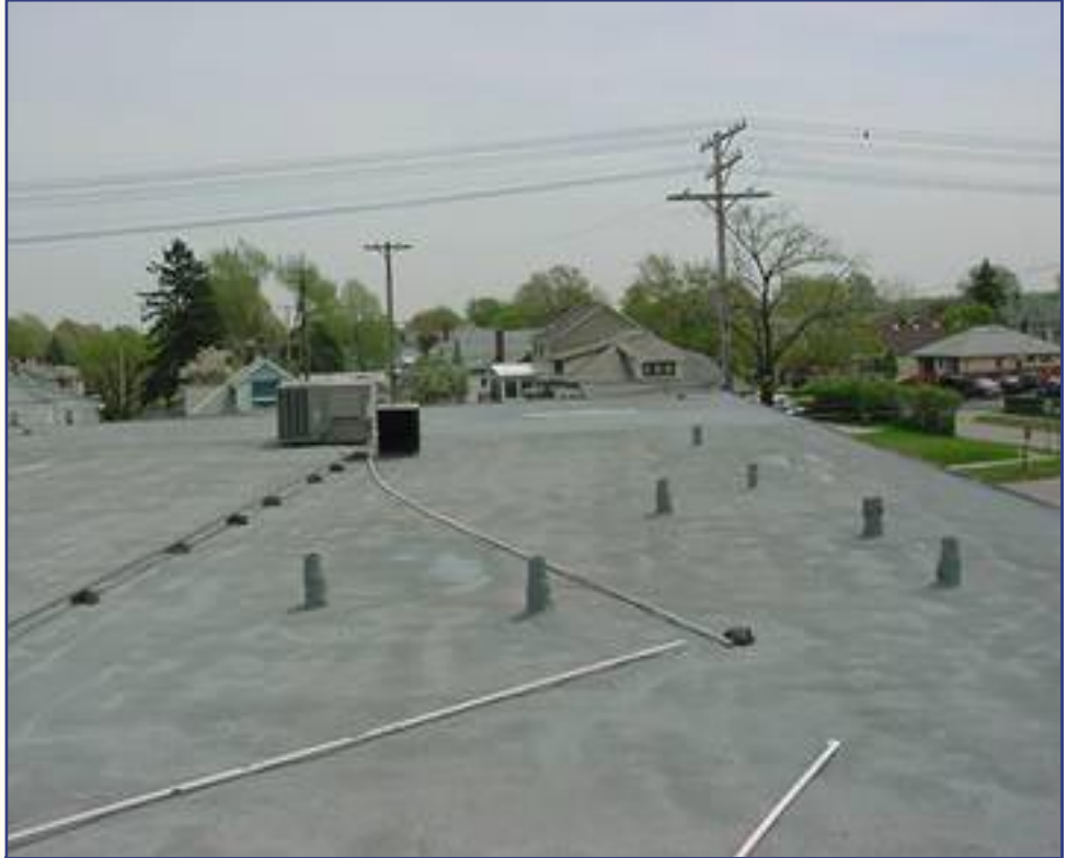
This 33,400 sq. ft. roof received a 10 year full system contractors warranty.
